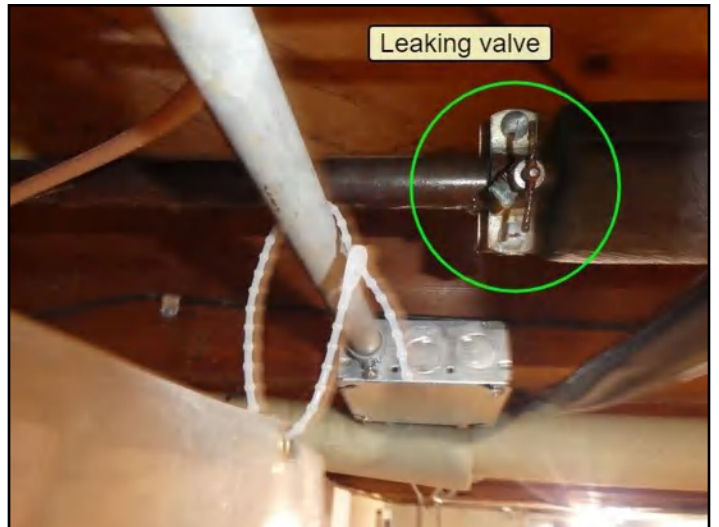
72. Leaking valve
