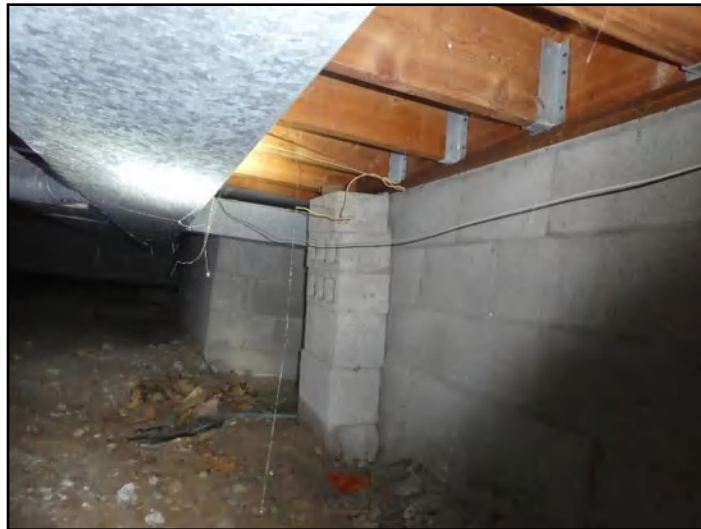
141. Improper support
