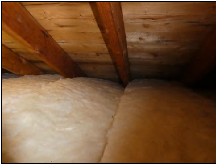
66. Missing baffles
