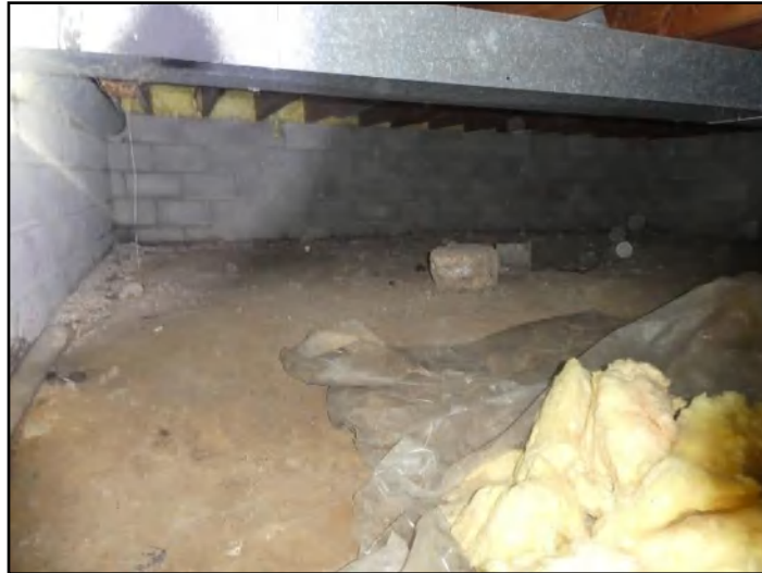
136. Dirt floor in crawl space
