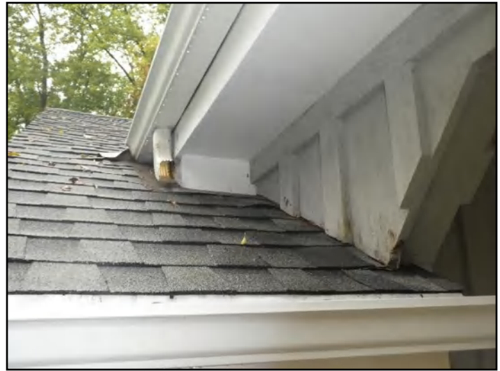
12. Discharge onto roofs
