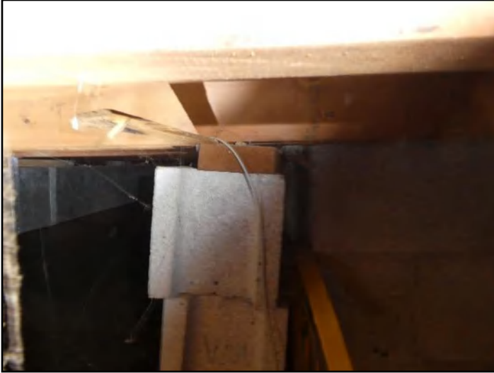
54. Improper support
