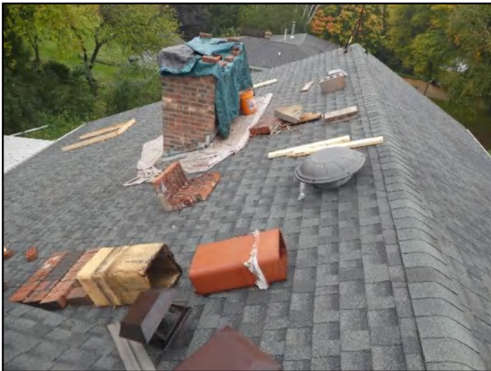
60. Chimney rebuild
