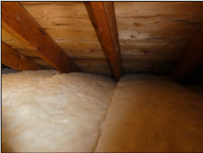
164. Missing baffles
