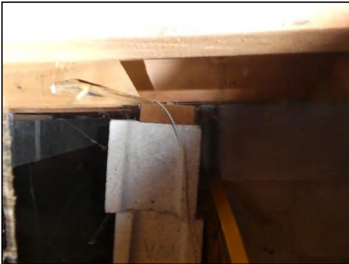
139. Improper support
