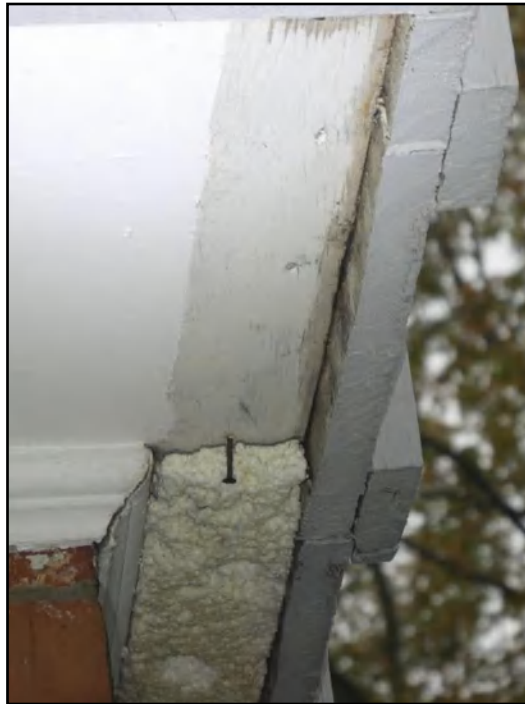
104. Visible insulation
