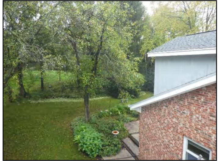
37. Trees to close to house. Trim back.
