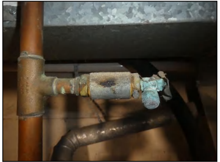
70. Leaking valve
