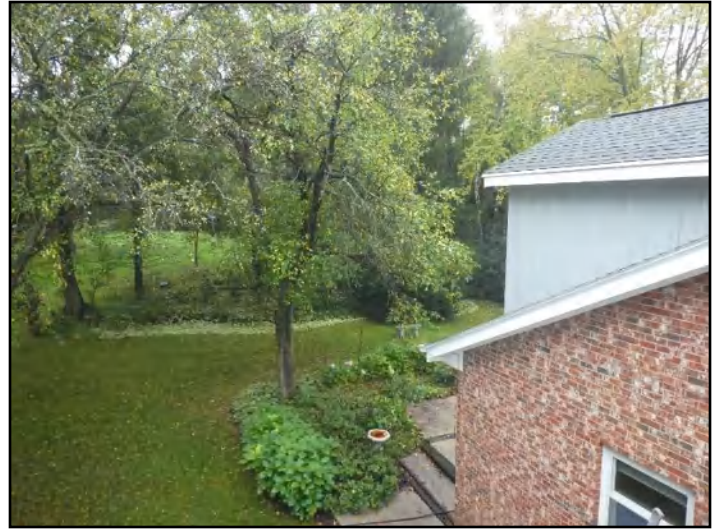
120. Trees to close to house. Trim back.
