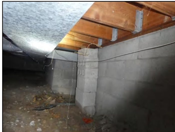
56. Improper support
