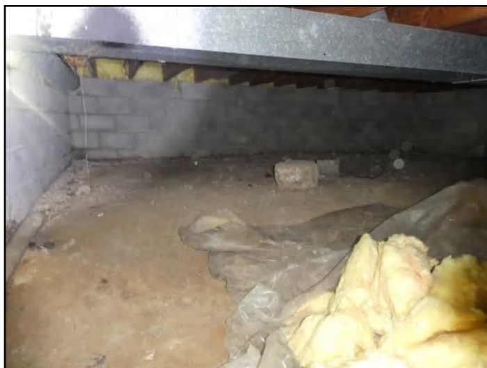
53. Dirt floor in crawl space
