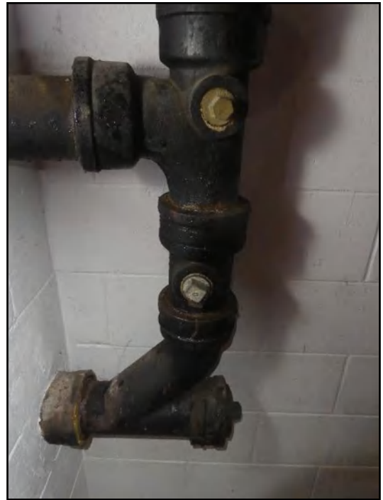
175. Cast iron main stack
