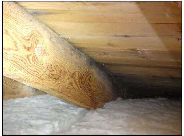
67. Missing baffles
