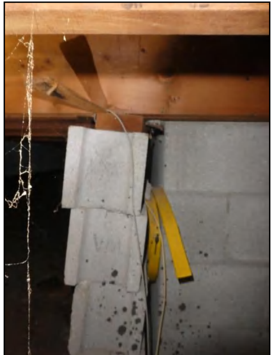
140. Improper support
