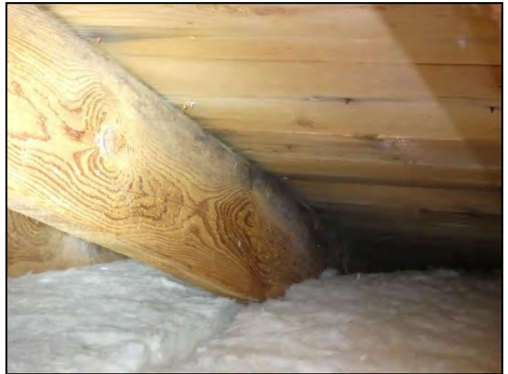
165. Missing baffles
