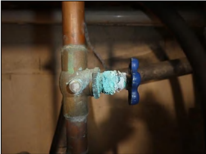
168. Leaking valve
