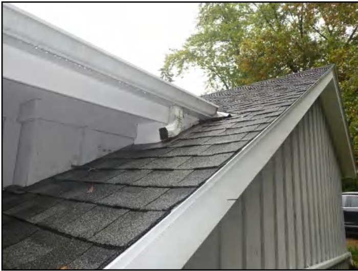
11. Discharge onto roofs
