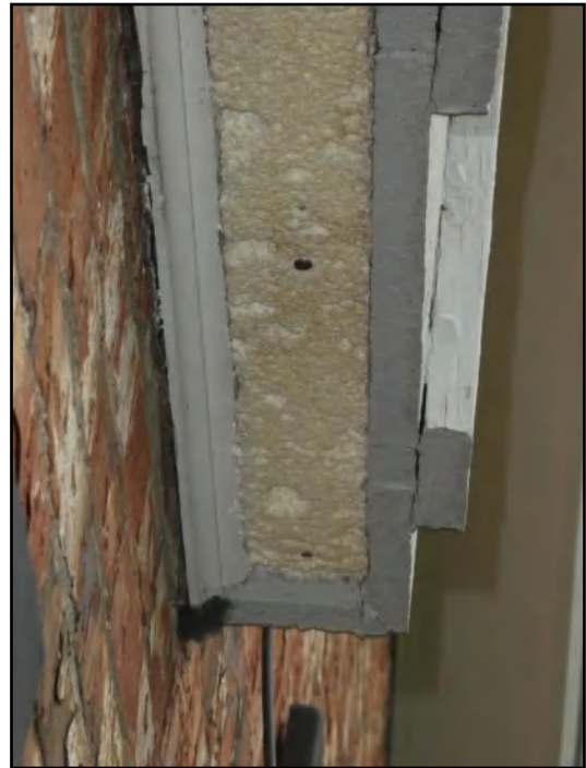
15. Visible insulation
