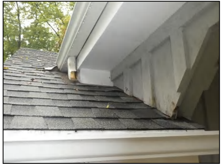
95. Discharge onto roofs
