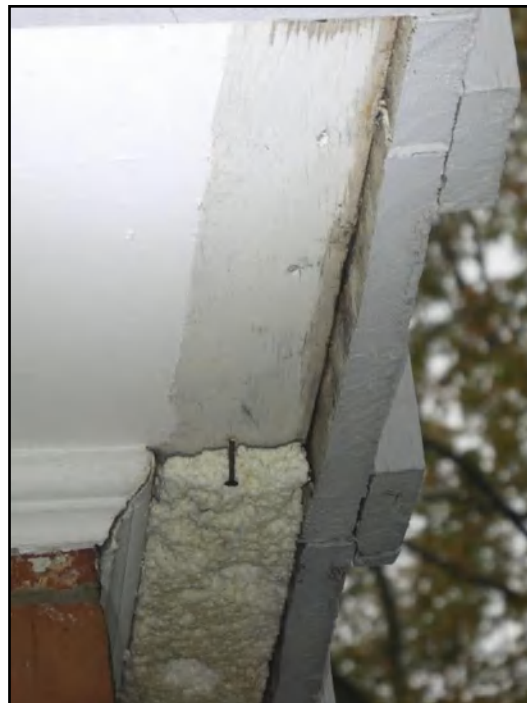
16. Visible insulation
