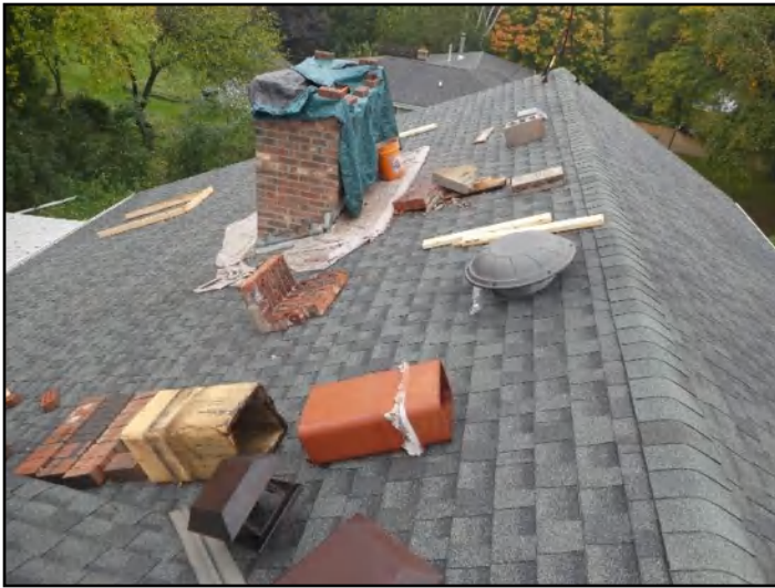
149. Chimney rebuild
