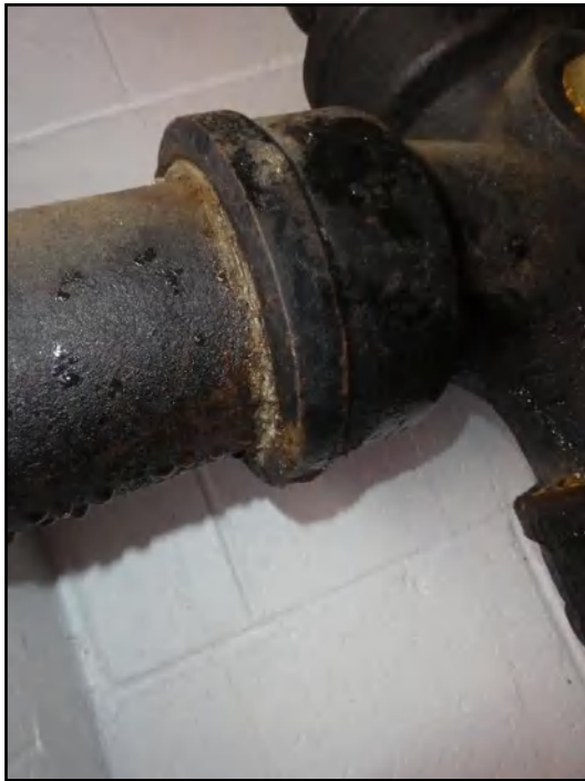
75. Cast iron main stack
