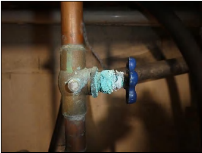
69. Leaking valve
