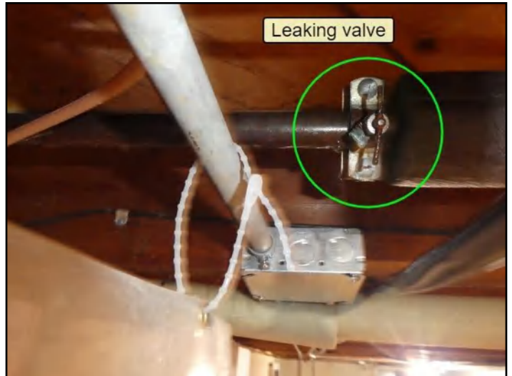
171. Leaking valve
