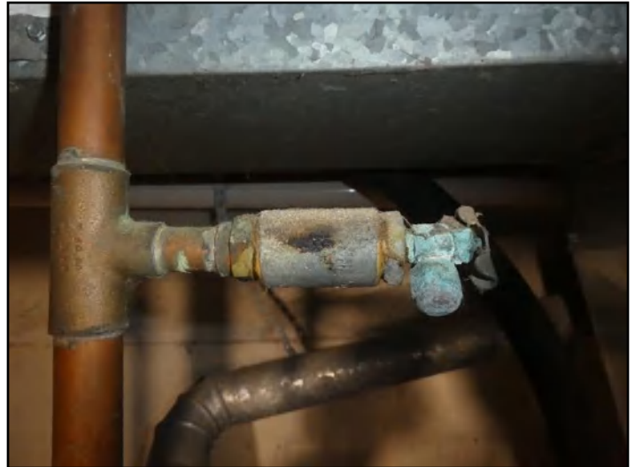
169. Leaking valve
